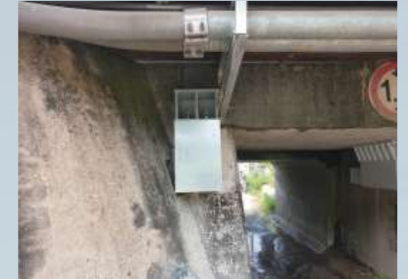
After shear key construction
