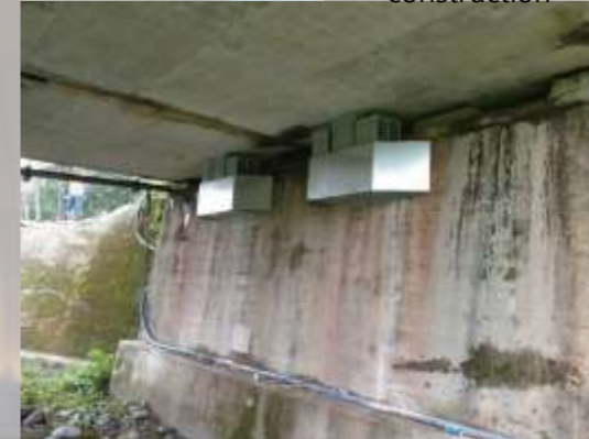
After RC SLAB construction
