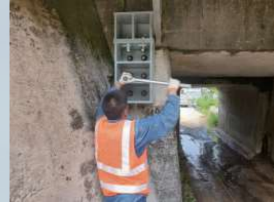
Shear key under construction
