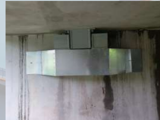
RC SLAB construction photos
