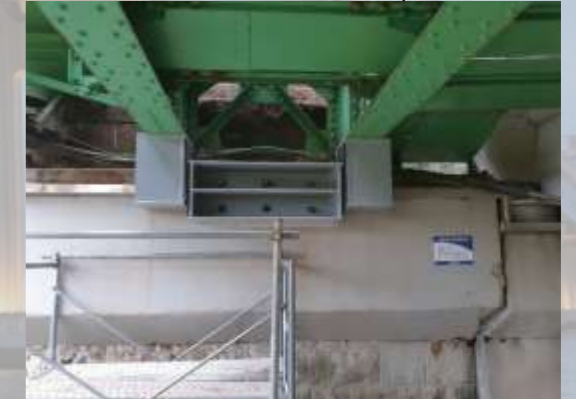
Plate girder bridge construction photos
