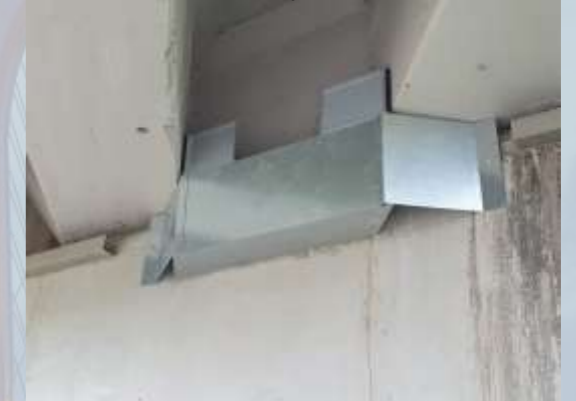
T-BEAM construction photos
